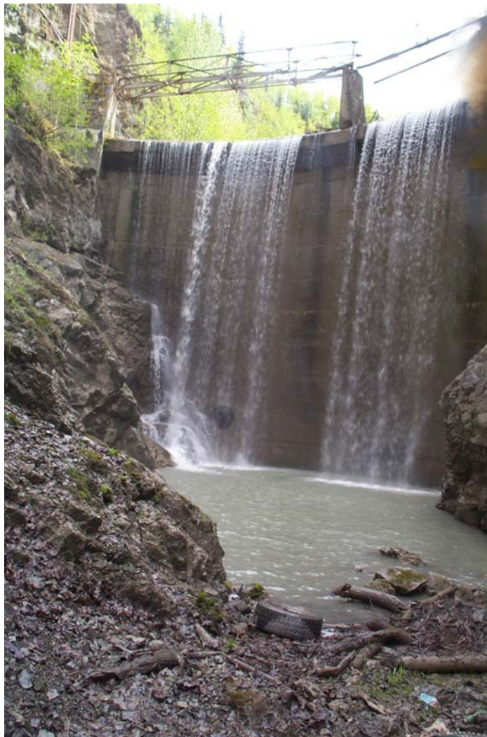
Photo 1: Backfilled Lower Eklutna Dam
